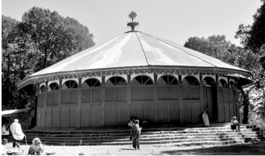
Fig. 10: Exterior of Däräsge Maryam church
